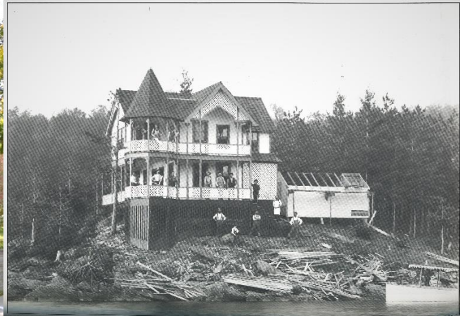
Seldoncliffe (under construction) Muskoka cottage
